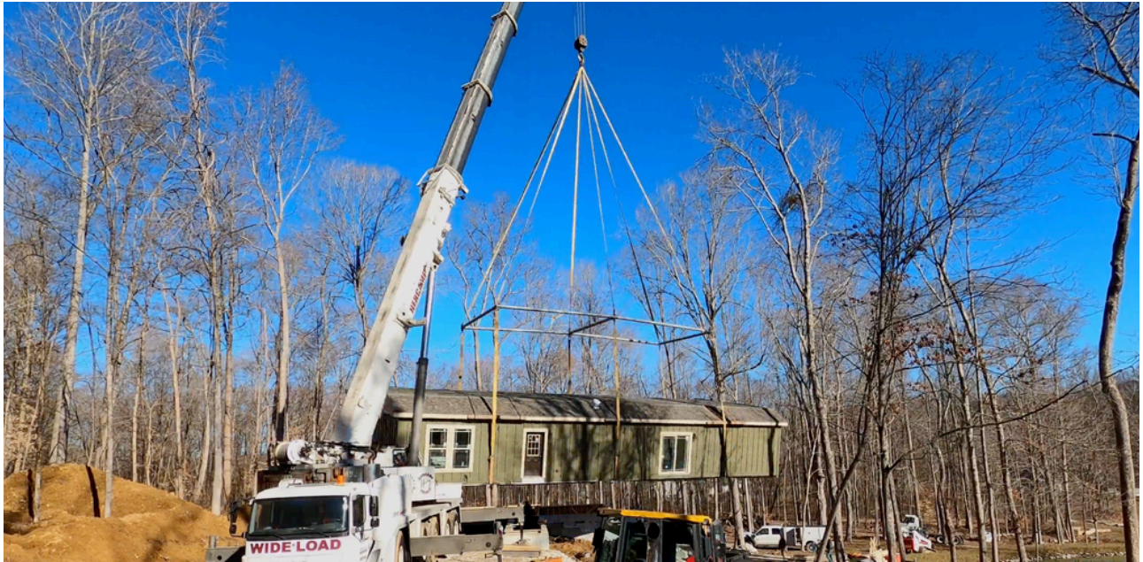
Setting a modular home by crane on a Florida homesite. (Photo: Florida Manufactured Housing Association)
